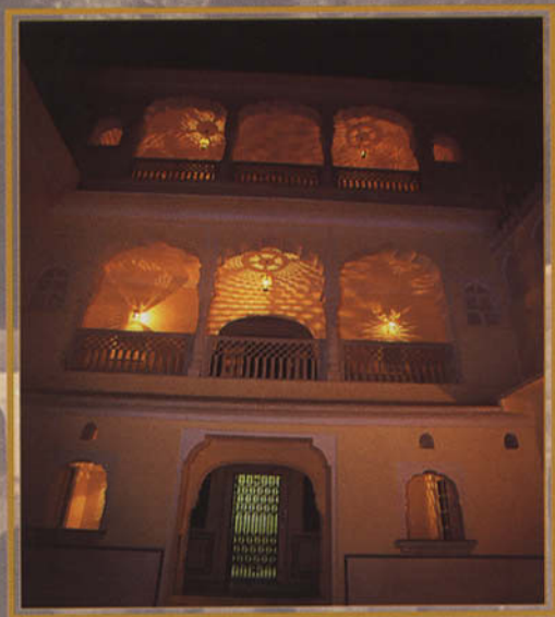
The Lift Facade
